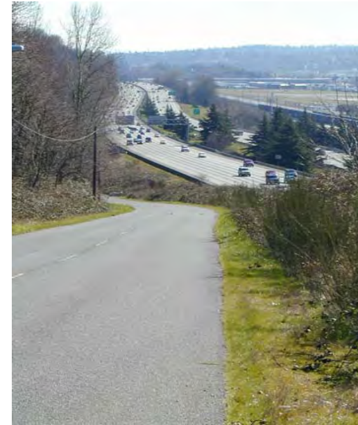
Military Road crossing under I-5
