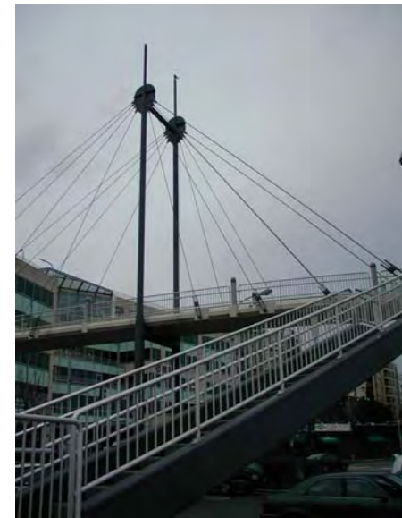
Galer Street Pedestrian Bridge
