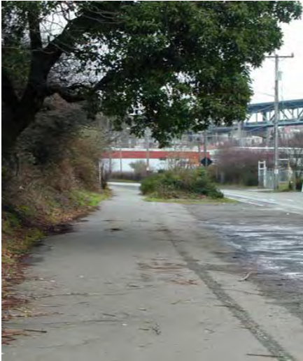
Abandoned trail on North Lake Avenue
