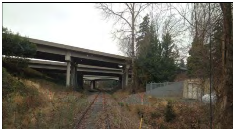
Exhibit 12. ERC passing under I-405 at the Interchange with SR-520
