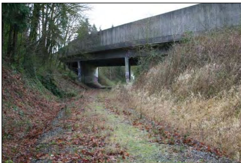
Exhibit 13. Wilburton Tunnel Crossing
