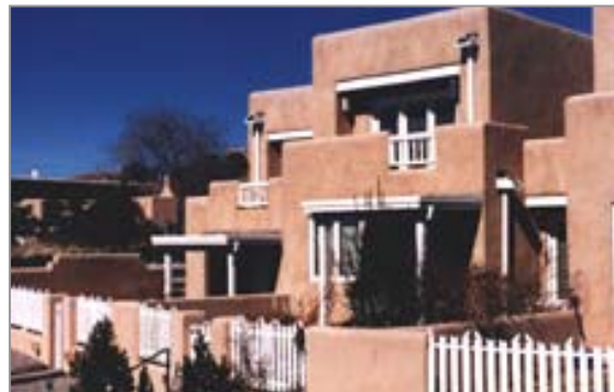
Pueblo Hermosa, a Santa Fe, New Mexico Housing Authority affordable ownership housing project, utilized a converted resort.
