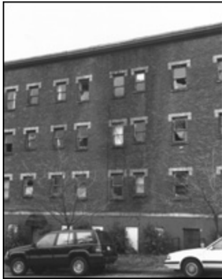
The Annobee's crumbling exterior before rehabilitation.
