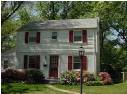
Affordable single-family home, Montgomery County, Maryland.
