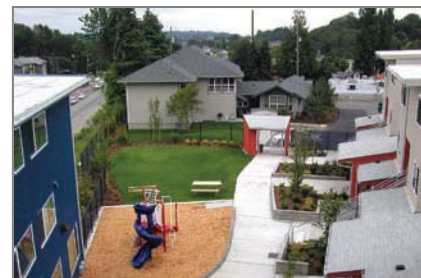
Name: Katharine's Place Type: New, multi-family construction. Square Feet: 32,040 Location: Seattle's Rainier Valley neighborhood.
