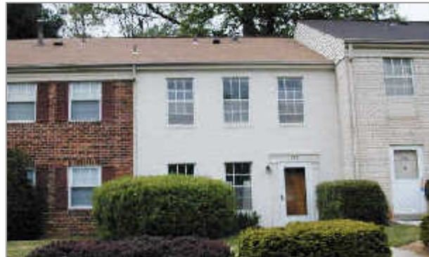
Single-family, affordable row housing, Montgomery County, Maryland.
